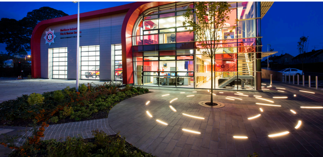
Omagh Firestation, Ireland
