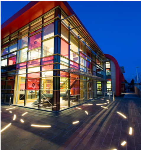
Omagh Firestation, Ireland
