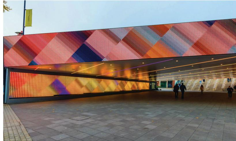
Within the ceiling, bespoke Light Lab products glowline, linear leds (also SPI-controlled), link the two walls, completing the "crossover" effect. Intelligent lighting control is provided by the pharos lpc100 controller.
